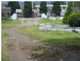
Poor condition of school entrance
